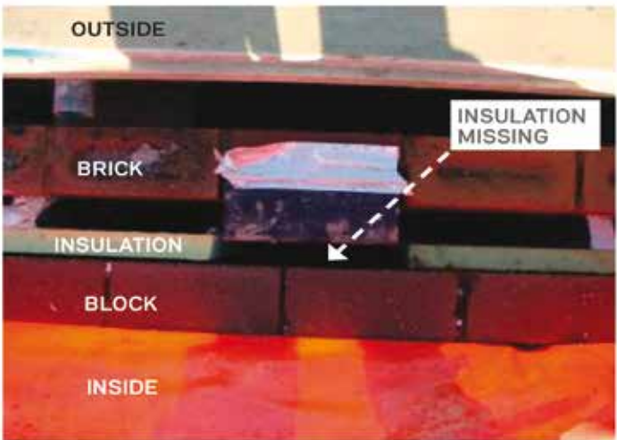
PLAN OF SUB FLOOR VENT BLOCKING INSULATION
