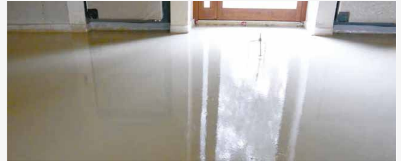
Machine application of the self-levelling screed on an old concrete substrate
