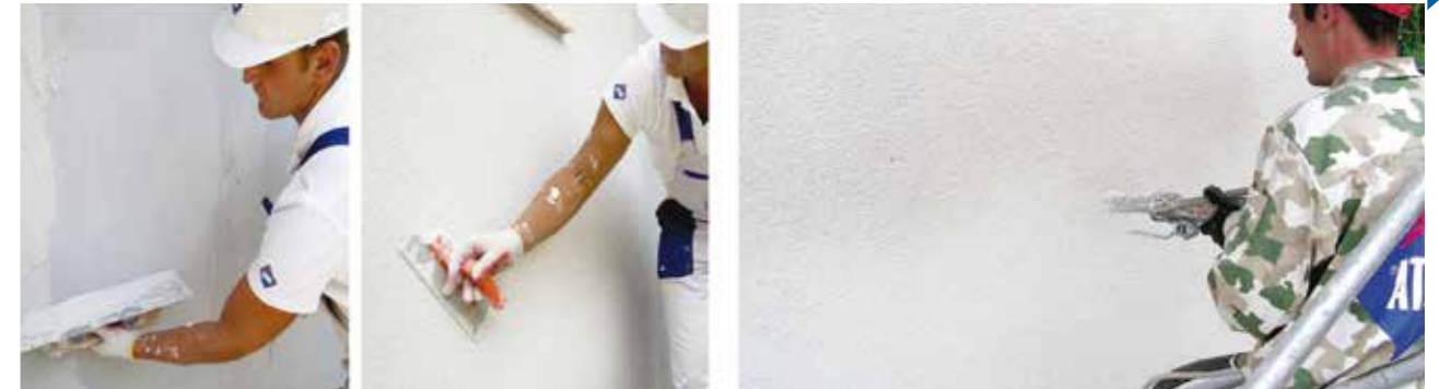
Applying renders using a steel trowel
