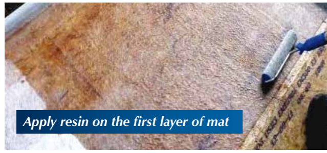
Apply resin onto deck
