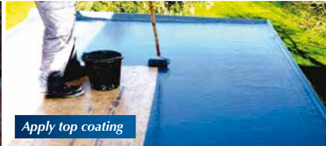
Continue overlapping each strip by 50 mm
