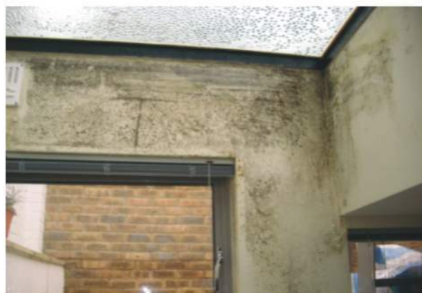
Photo1: Typical moulds (Aspergillus Niger) and fungus in new flat LONDON, February 2008
