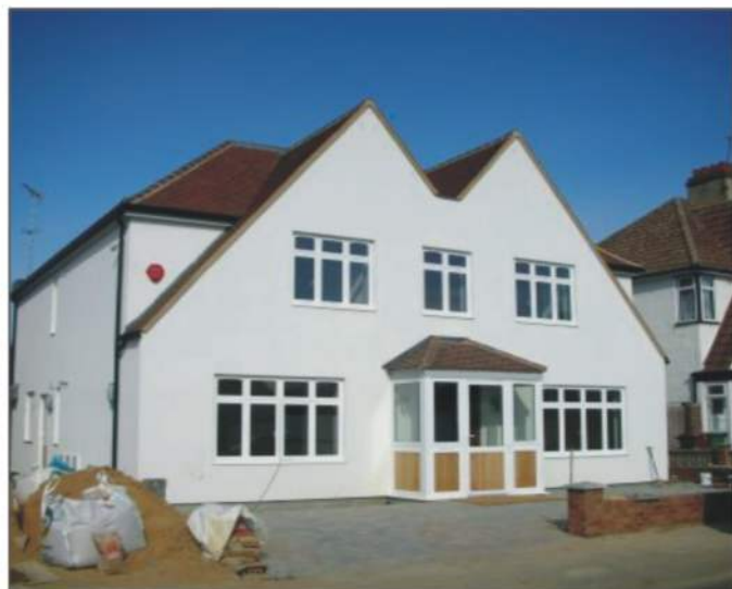
detached house in south London- fine layer render with external wall insulation system
