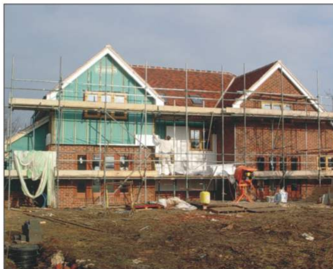
detached house near Stansted, 'old' brick plus render with external wall insulation system
