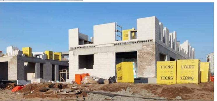
**YTONG 3,6 Standard Blocks** - perfectly suited to build the internal and external leafs of cavity walls, solid walls, separating walls, partitions, flanking walls, soil conditions D S-1. Available in range of thicknesses. Laid weight for design purpose incl. 3% moisture approx. 485 kg/m³.
