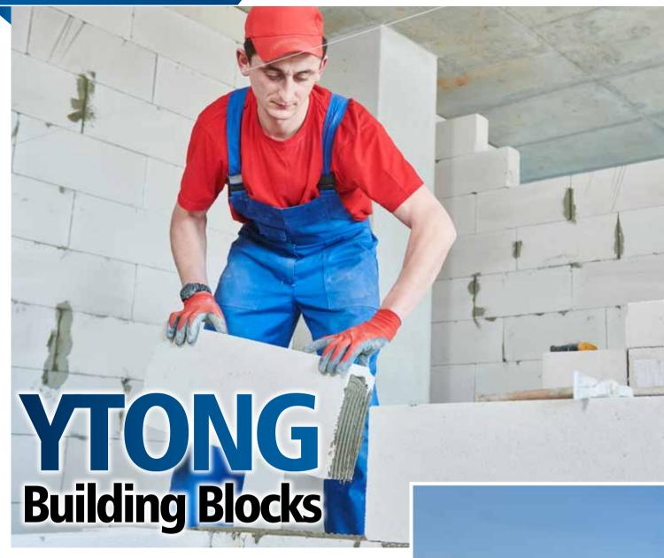
Ytong aerated concrete building blocks are used for internal partition walls and load bearing external walls constructions. Ytong blocks can be laid in either standard mortar or thin layer mortar. Any mortar used should comply with BS EN 998-2 specification for Mortar for Masonry. Ytong blocks is a thermal efficient option due to their insulating properties. The dimensional accuracy of Ytong blocks make them perfect choice for thin joint system. Moreover, Ytong blocks are highly sustainable.
