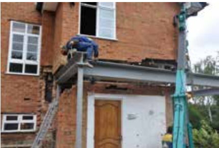
Bolting beams
