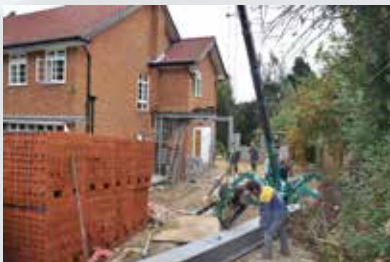
Steel installation
