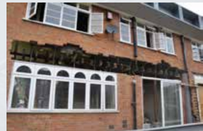
Propping existing structure
