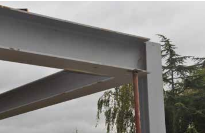
Steel beams connection
