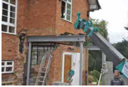
Installing steel beam
