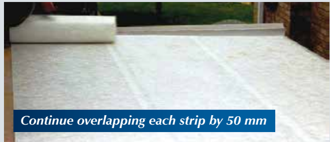
Lay out first strip of mat along lowest point
