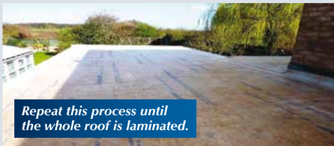
Apply resin on the first layer of mat
