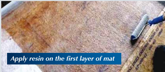
Apply resin onto deck
