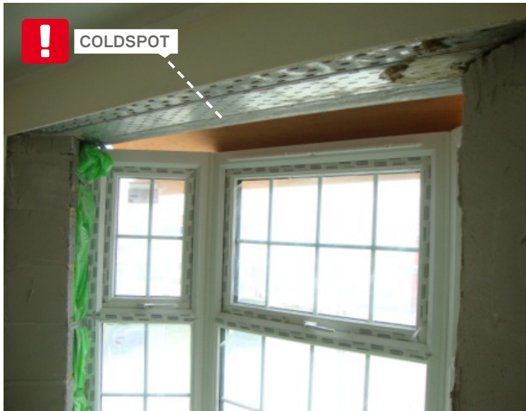
THICK FRAME AND POSTS INCREASES HEAT LOSS
