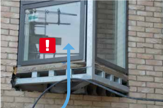
CONTINUOUS STEEL CREATES COLD BRIDGE
