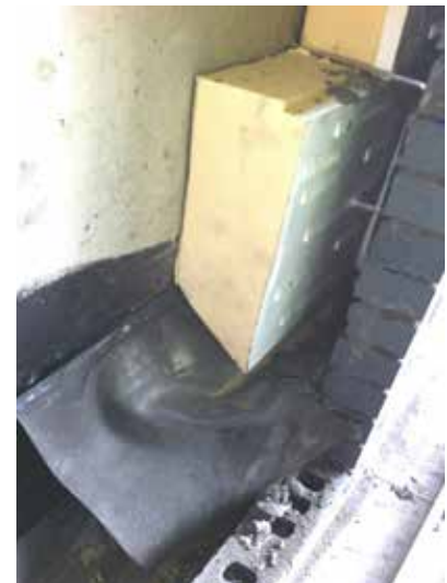
CUT INSULATION AROUND CAVITY TRAY
