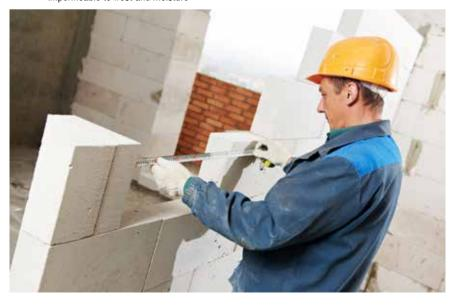
**YTONG 3,6 Standard Blocks** - perfectly suited to build the internal and external leafs of cavity walls, solid walls, separating walls, partitions, flanking walls, soil conditions D S-1. Available in range of thicknesses. Laid weight for design purpose incl. 3% moisture approx. 485 kg/m³.
