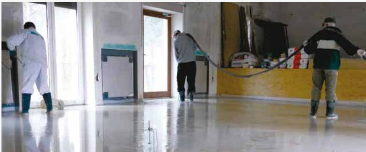
Machine application of the fast-setting anhydrite-based screeds is a perfect solution for large surfaces (over 15 m 2 )
