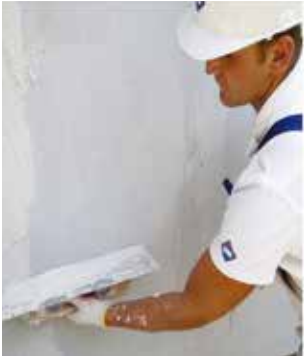
Applying renders using a steel trowel
