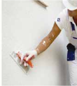
Applying renders using a steel trowel
