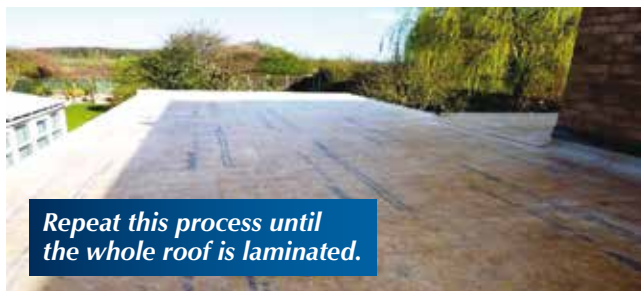
Apply resin on the first layer of mat
