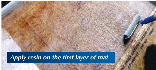
Apply resin onto deck
